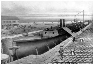
damage the MERRIMACK's engines or completely destroy her hull, as well as not ensuring the dry dock's destruction allowed the Confederates to utilize both to create the world's first iron-clad; the CSS VIRGINIA, shown here in the dry dock in early 1862.
